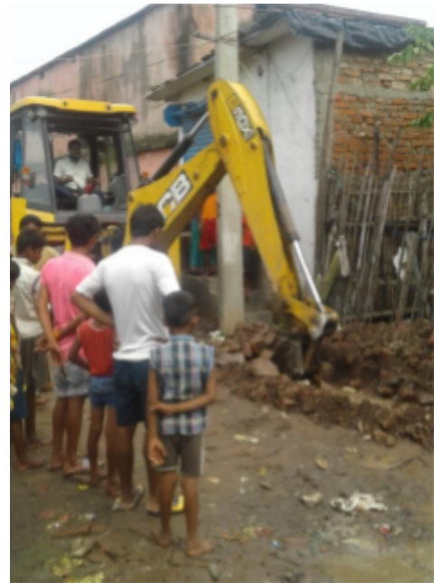
Figure 2- Excavation work for the drainage network has taken place.
